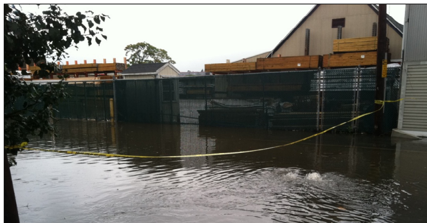
Figure 8 POST-HURRICANE FLOODING NEAR AN EAST COAST LUMBER STORAGE FACILITY
